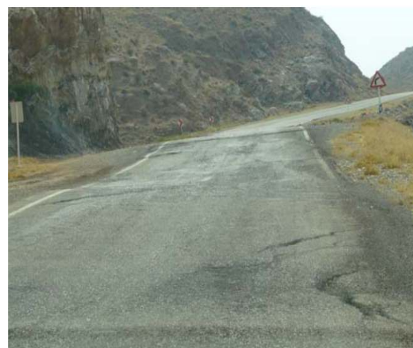
Fig. 6-29. Road from Darreh-Shahr to Abdanan (32km from Darreh-Shahr): Fissures and land subsidence caused by the 18 August 2014 earthquake (about 42km distance to epicenter).
