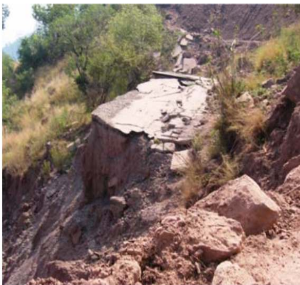
Fig. 6-15. Islamabad–Muzaffarabad road destroyed by Balakot earthquake on 8 Oct. 2005
