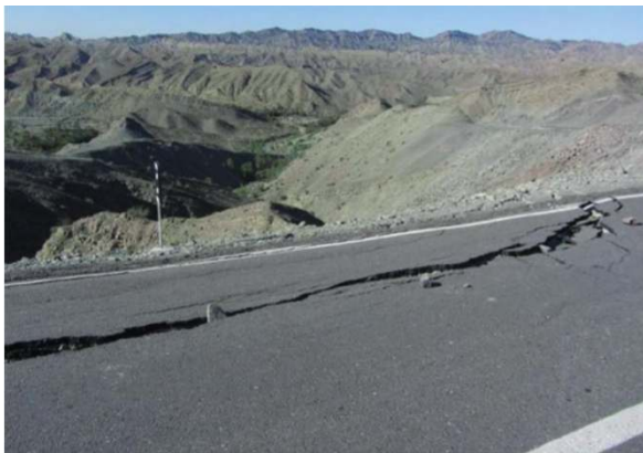
Fig. 6-23. The tension cracks in the Goharan to Irar road, created during the mainshock of the 11 May 2013 earthquake.
