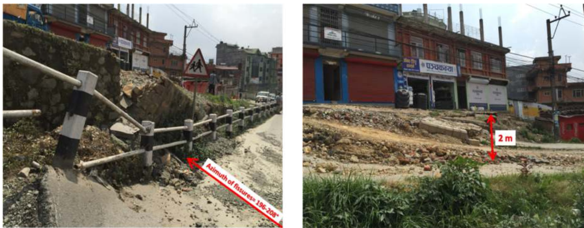
Fig. 6-21. Ground surface fissures with azimuth of 196-208° and 2m vertical displacement occurred in the road between Bhaktapur and Kathmandu.
