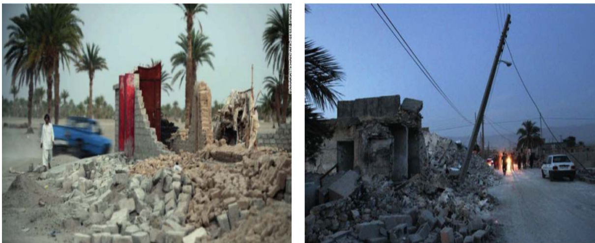
Fig. 6-4. The damages in the epicentral region of Gosht, Saravan Earthquake, 16 April 2013, Mw7.8 earthquake (Photo by AFP).
