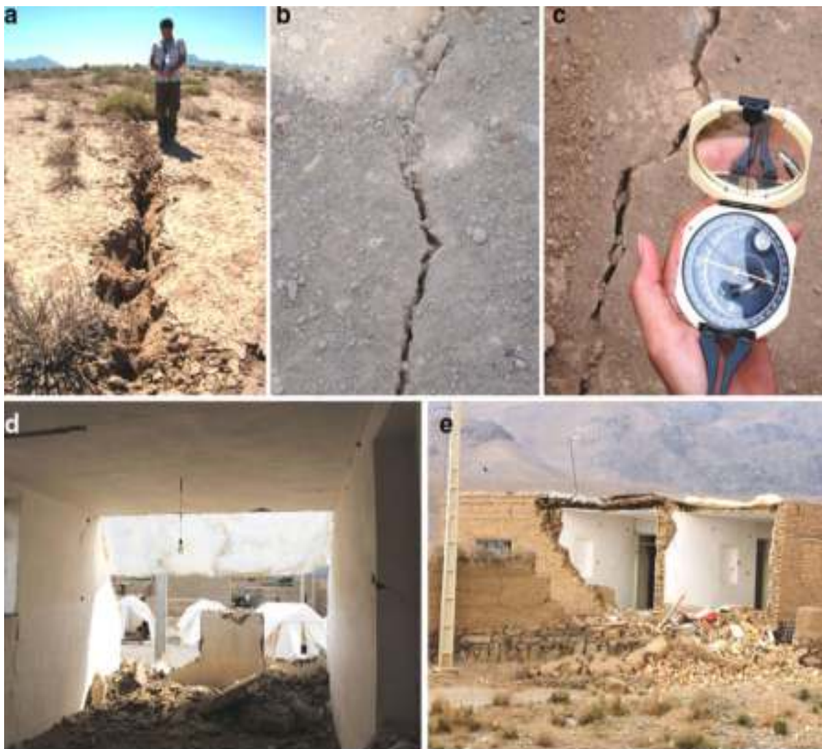
Fig. 6-8. Field photographs: a Coseismic fracture near the epicenter (Foroutan et al. 2010). b Crack from the 2010 Kuh-Zar earthquake (near the epicenter), cracks strike E to W. c Fissuring in Kelu village, 5 kilometers from the epicenter, crack strike is N70. d Typical adobe-brick house at Kelu; the non-load-bearing walls collapse in an earthquake first. e Collapse started in the corner, where it was easier to initiate instability.
