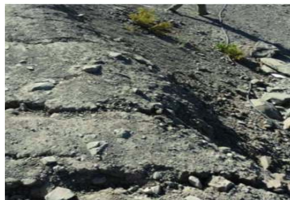
Fig. 6-24. Surface fissures in the epicenter of 11 May 2013, Mw6.2 Iran earthquake (in the village of Irar).
