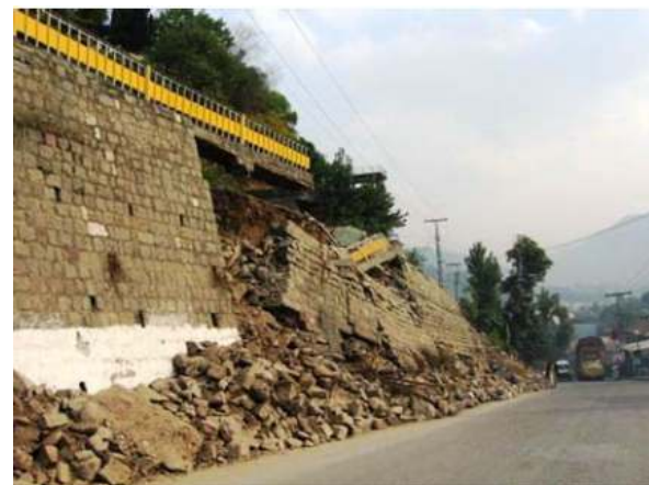
Fig. 6-11. Muzaffarabad: the retaining wall collapse due to Balakot earthquake mainshock on 8 Oct. 2005
