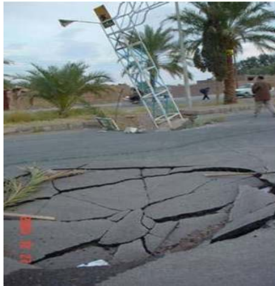
Figure 6-27. The sinkholes created during the 26/12/2006 Bam earthquake in Baravat.
