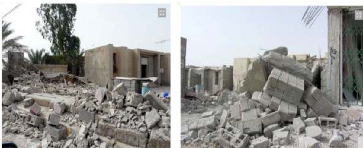
Fig. 6-5. Buildings damaged in the 2013 Mw6.4 Shonbeh (Bushehr), Iran earthquake
