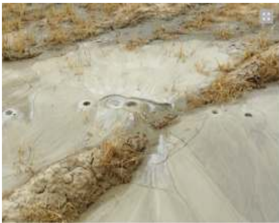
Fig. 6-30. Close-up view of liquefaction in the Dashte Zaal area.
