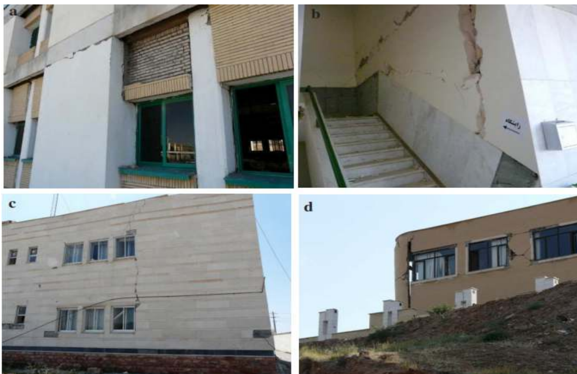
Fig. 6-7. (a and b). Examples of Heris Hospital, (c and d). Example of diagonal cracks in walls, and of slight structural damage in the region, respectively (Zaré, 2012).
