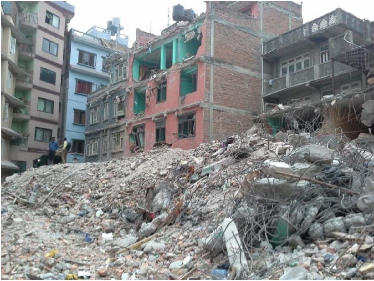
Fig. 6-1. Sever damages to the building in the Dhading New Bus Park in Gongabu Ring Road northwest of Kathmandu.
