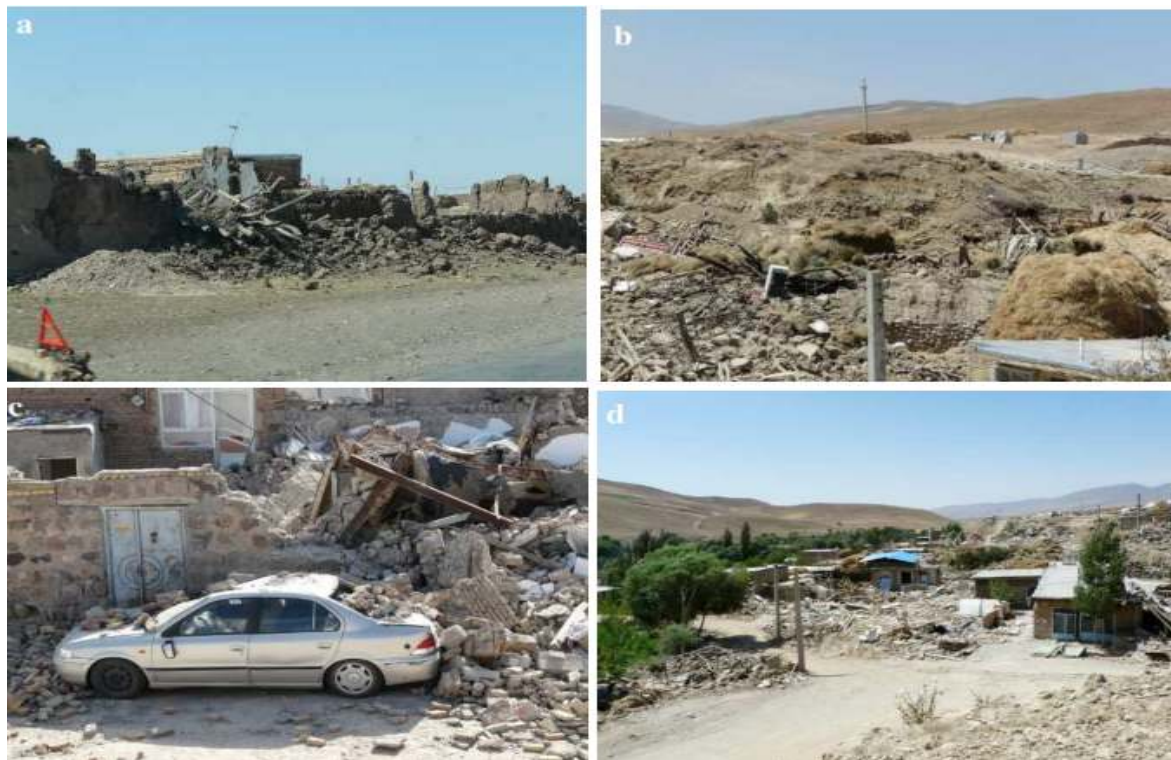
Fig. 6-6. (a and b) Examples of total collapse in very weak buildings, (c and d). Examples of demolished buildings in Varzeghan (left-c) and Baj e Baj (right-d) (Zaré et al, 2012).
