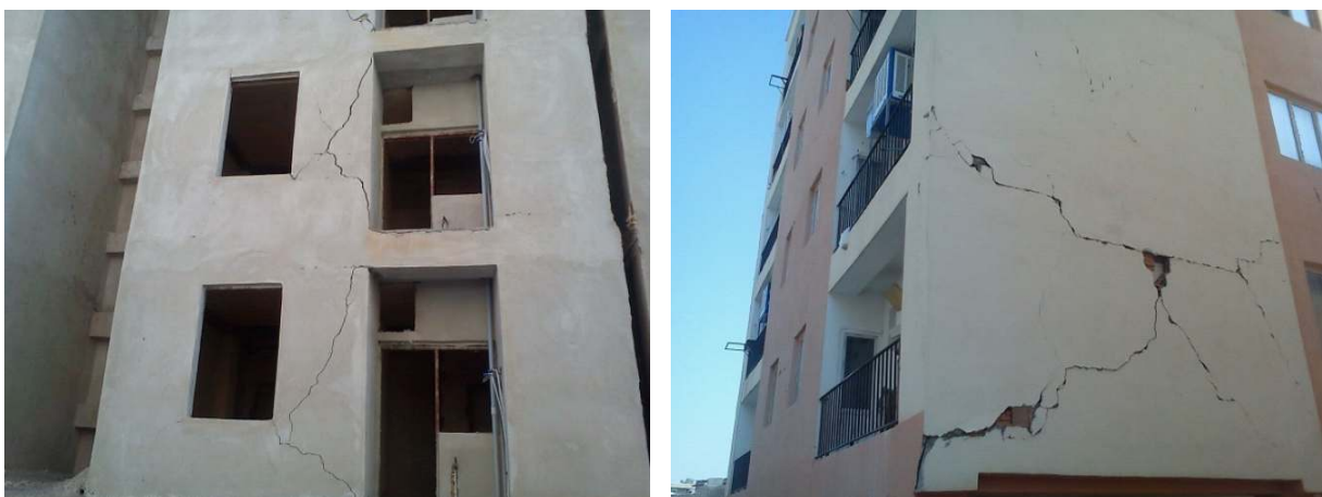
Fig. 6-3. Fissures created in "Mehr" Apartments (Maskan-e Mehr) in Abdanan (38km to the epicenter); constructed about one year ago and suffer extensive damages due to an intensity VI (EMS98) in the 18 Aug 2014 Mormori earthquake.
