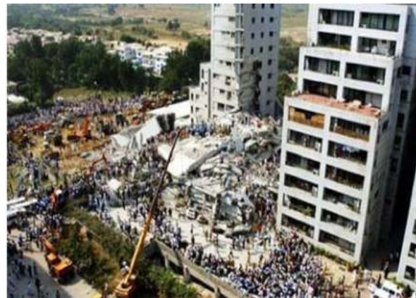
Fig. 6-13. Margala Tower collapse in Islamabad (Associated Press, Oct. 2005)
