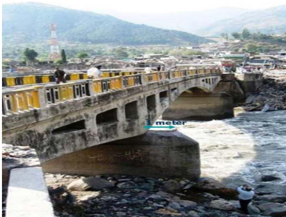
Fig. 6-10. About 1 m displacement in the abutment of Balakot southern bridge due to the earthquake mainshock on 8 Oct. 2005
