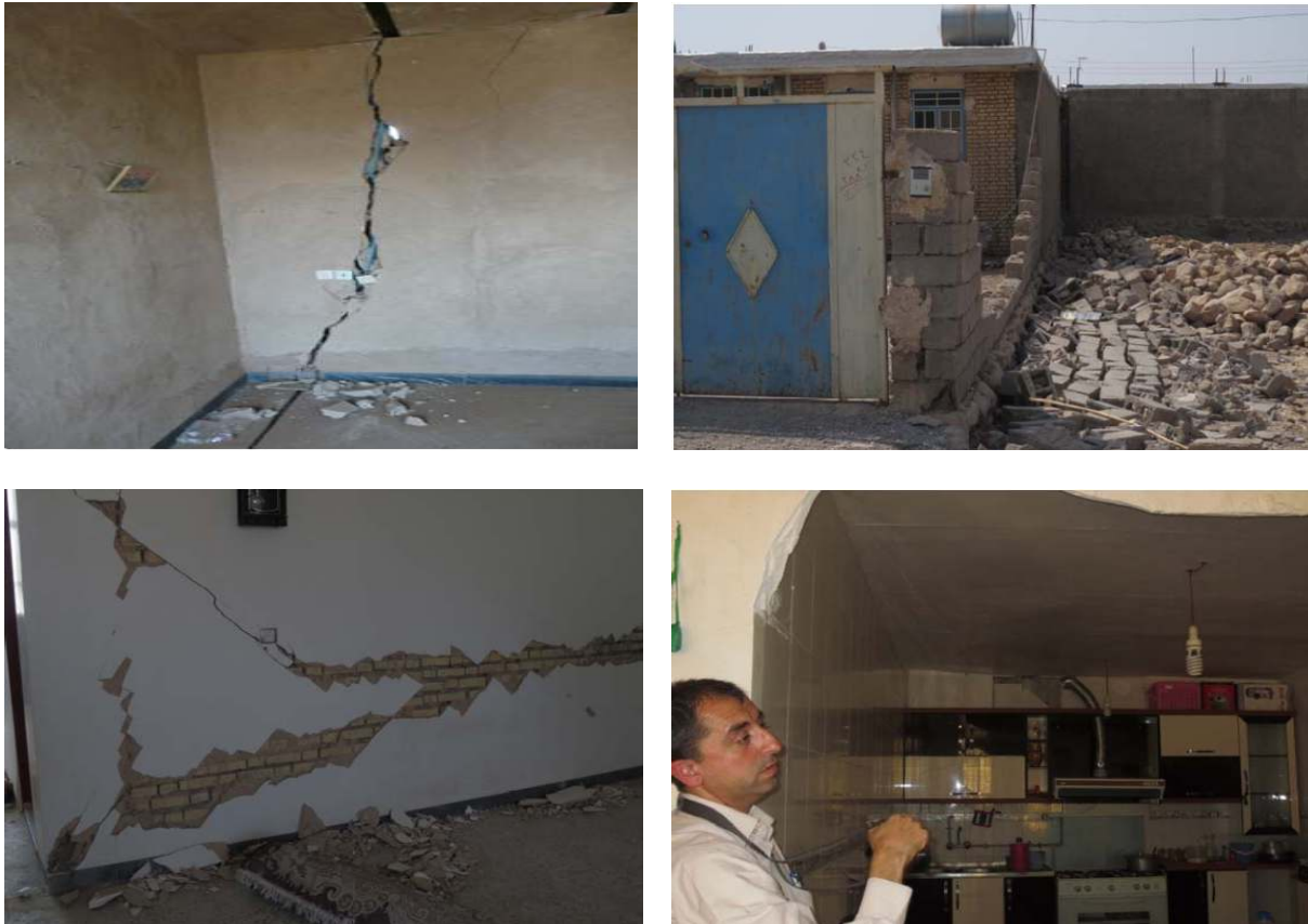
Fig. 6-2. Damage to the buildings in Abanar: collapse of walls, figures and object and plaster fall.
