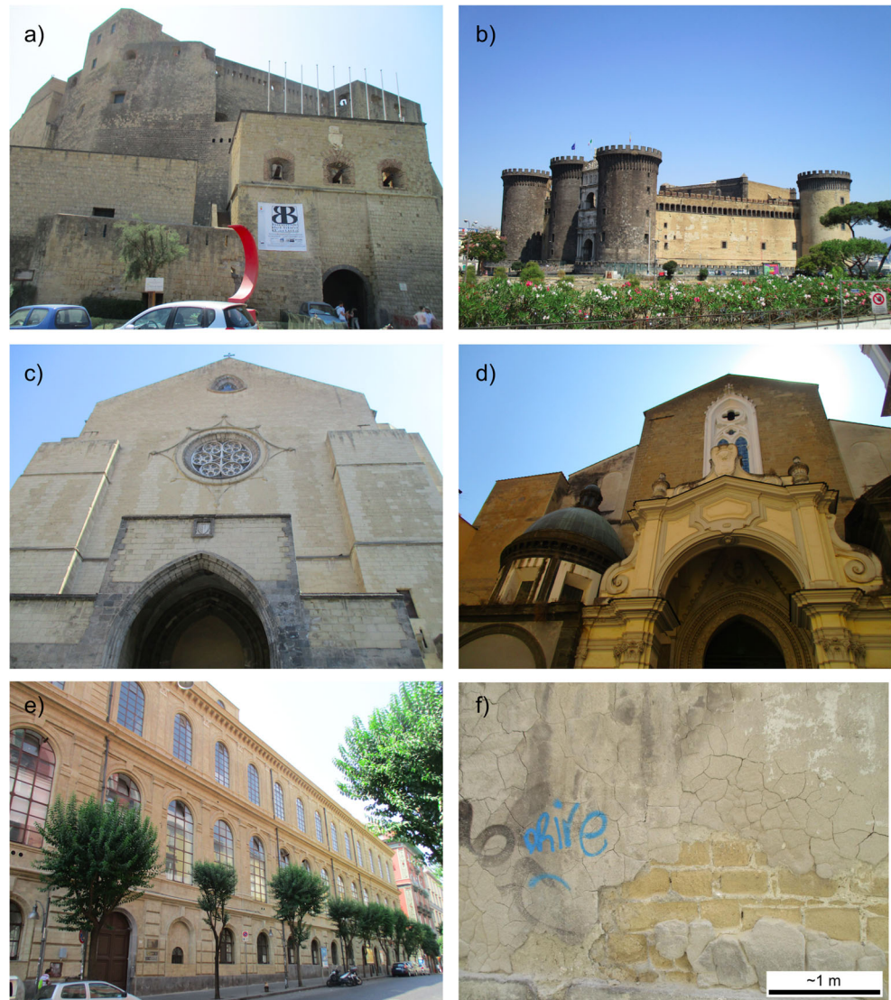
Fig. 2 Photographs of buildings constructed using Neapolitan Yellow Tuff (NYT) in Naples. (a) Castel dell'Ovo, (b) Castel Nuovo, (c) the church of Santa Chiara, (d) the church of San Domenico Maggiore, (e) the Academy of Fine Arts, and (f) a plastered wall constructed using NYT within the ancient city centre of Naples
