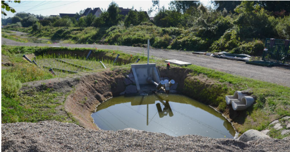
Fig. 4 Hybrid treatment system just after construction. The settling pond is on the lower side of the picture; the constructed treatment wetland is on the upper left side of the picture. A bit further behind, a discharge pond can be seen ( Source ICube Laboratory)
