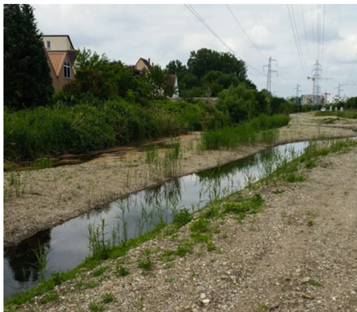
Fig. 3 Restored stream. A dead arm can be seen on the left side of the picture, and a meander on the right ( Source ICube Laboratory)
