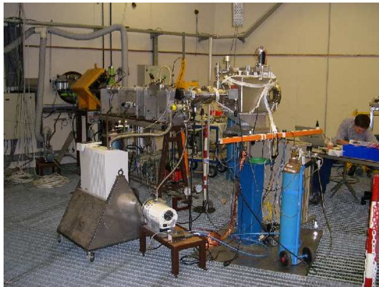
Figure 6.3: The SLIM beam monitor and related equipment installed in one of the extraction lines of the JRC cyclotron.
