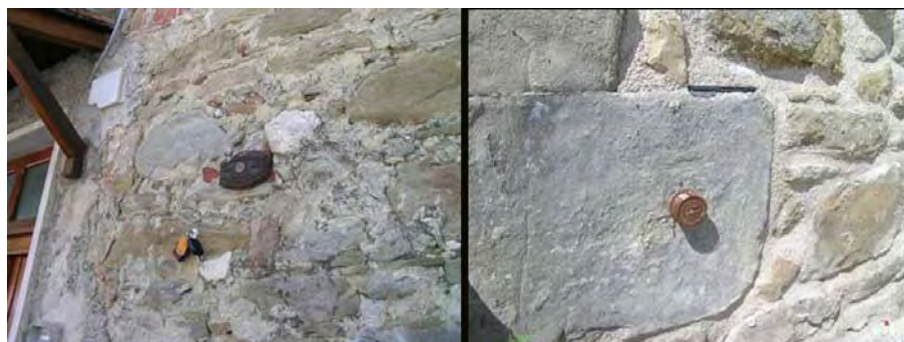
Figure 3.4. Typical benchmarks of the first order leveling Line 124
