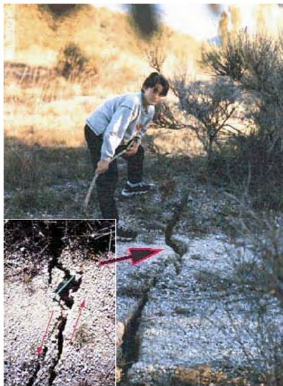
Figure 4.8. The 14 October 1997 rupture on the dirt road that takes to the Dominjianni house (courtesy of the Dominjianni family) and detail showing the presence of a left-horizontal component of movement.
