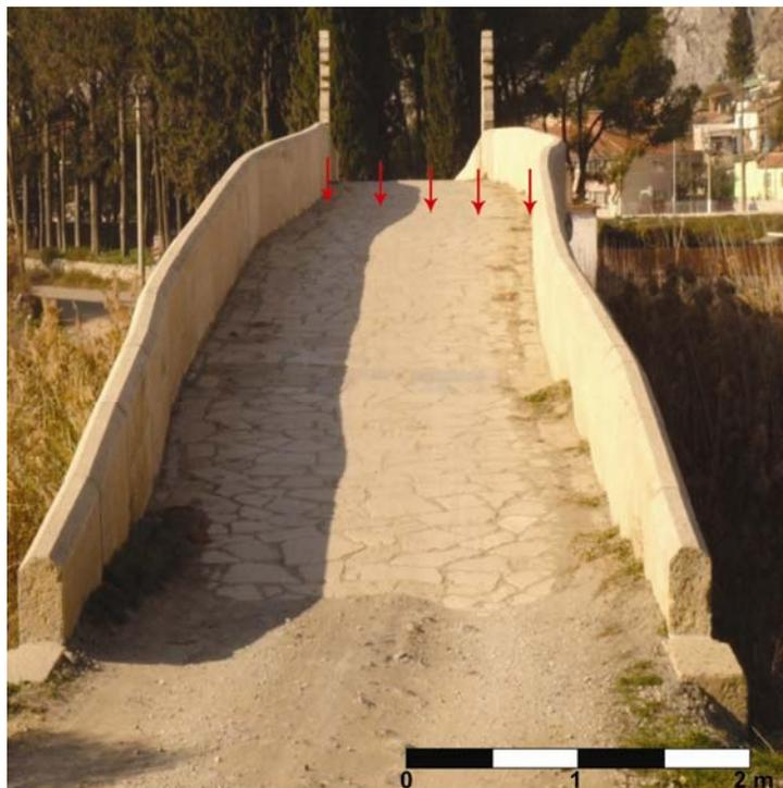
Figure 4.18: Sudden bending on the Ottoman bridge (~50 cm) pointed with red arrows (looking towards northwest).
