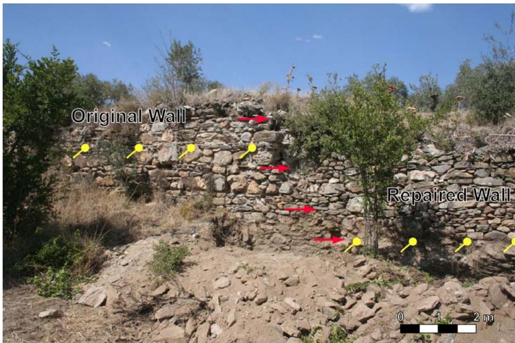
Figure 4.26: The Roman wall and its disturbed part (Yellow signs show the same stone level and red arrows indicate disturbed part of the wall).
