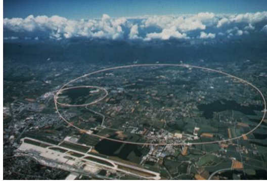
Figure 1.4: The bird's eye view of LHC at CERN.
