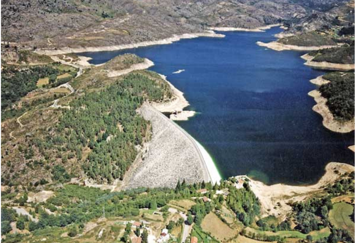
Figure 2.4: View of the Paradela dam.
