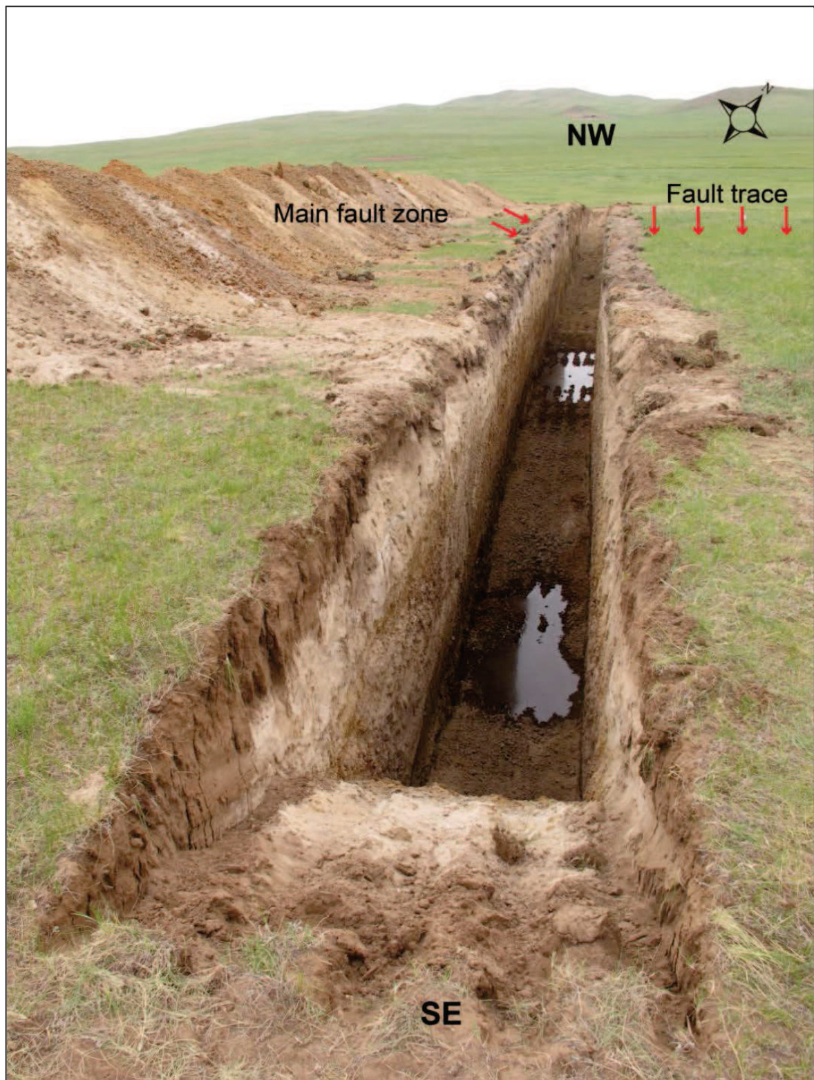
Figure 3-4: Muka-L trench (55 m long, 1 m width and 3 m deep) across the Sharkhai fault (red arrows). The fault zone is about 3m width and extends from the bottom of the trench up to the surface. We can see water at the bottom of trench, at 3 m deep, due to ice thaw.
