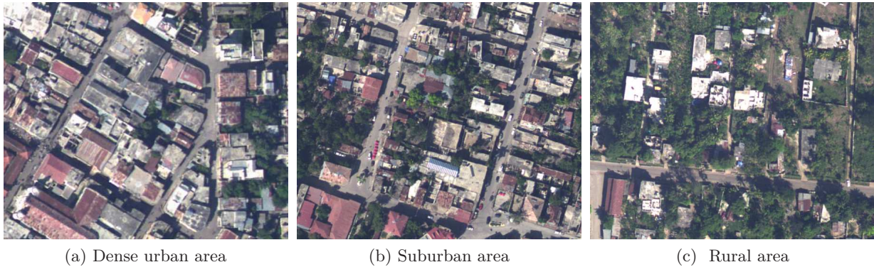
Figure 5.1: Different study areas: high dense urban area with very high population density and attached buildings, suburban area with residential trip and detached buildings, rural area with very low population density, detached buildings and high vegetation density
