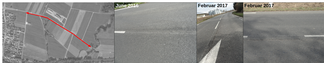
Figure IV.1.12: RD4: Crack at the centre line
