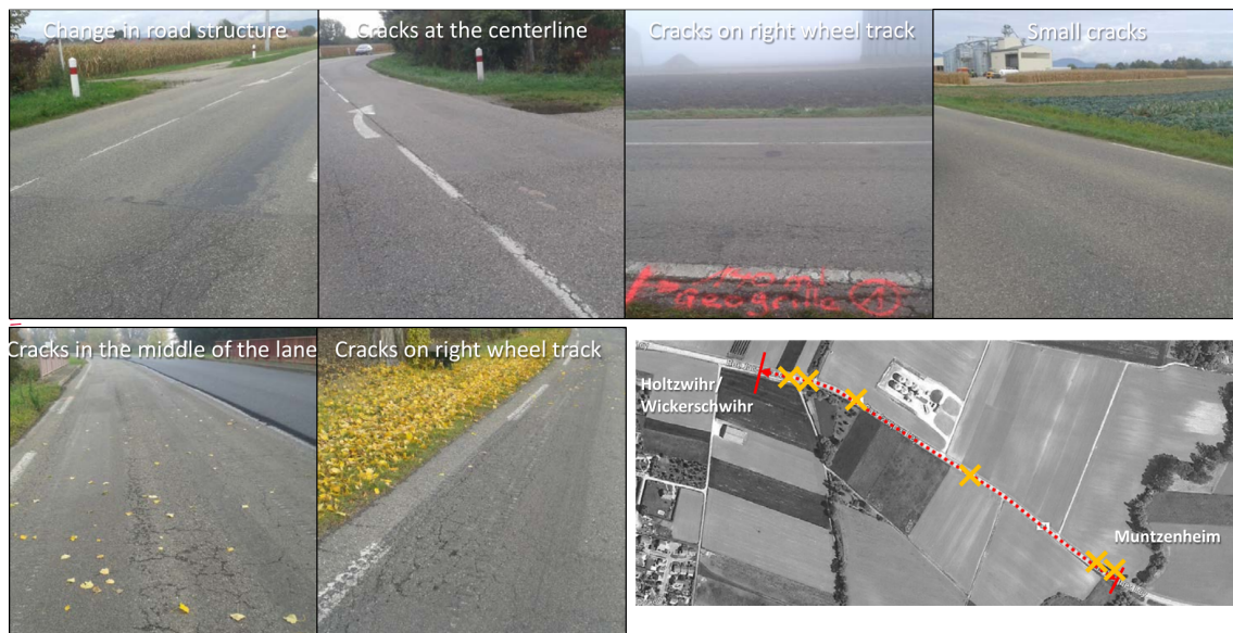
Figure IV.1.4: Photographs of the RD4 before maintenance and location of the pictures taken (map on the right, second line)
