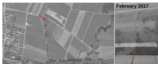
Figure IV.1.15: RD4: Crack between the section built in on 29/10/15 and the section built on 30/10/15
