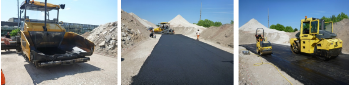
Figure III.1.3: Construction of lower layer: Finisher on unbound granular base course, test surface, compaction of the surface
