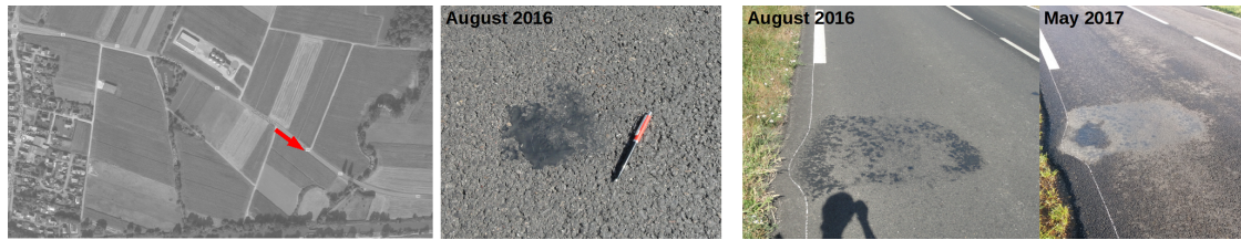
Figure IV.1.11: RD4: Medium and big bitumen accumulations
