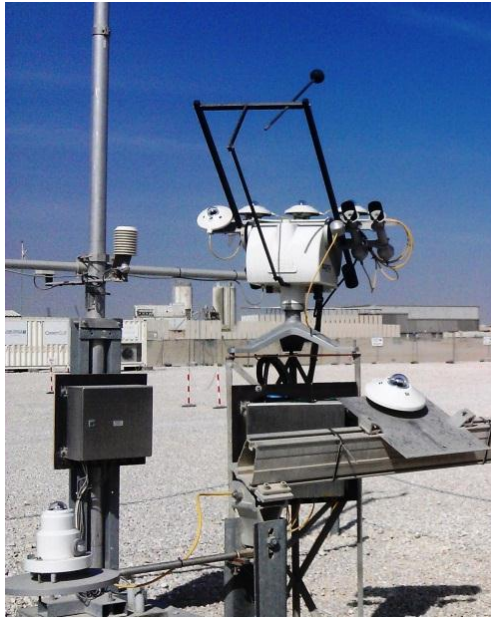
Figure 37. Weather station at the STF test site used to record wind speed and relative humidity. A separate, nearby particulate monitor was used for dust concentration measurements
