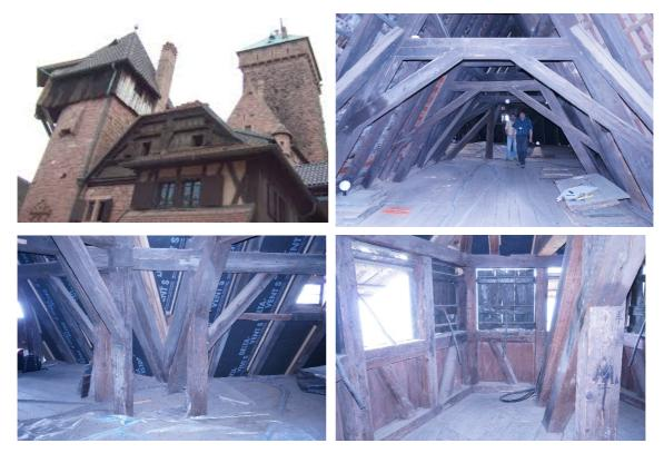
Figure 3.26. Castle of Haut-Kænigsbourg (top left) and details of its truss structure (top right and bottom).
