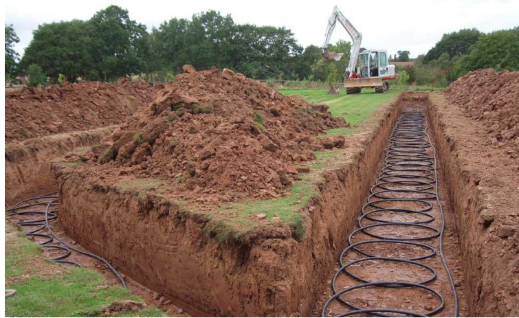
Figure I.12. The installation of a slinky-type HGHE (Pullen, 2019)
