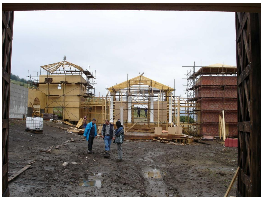
Figure 36: la construction du palais de César. ©Fathi Rached
