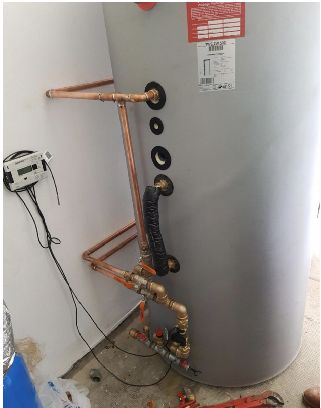
FIGURE 5.16: Photography of the newly installed boiler
