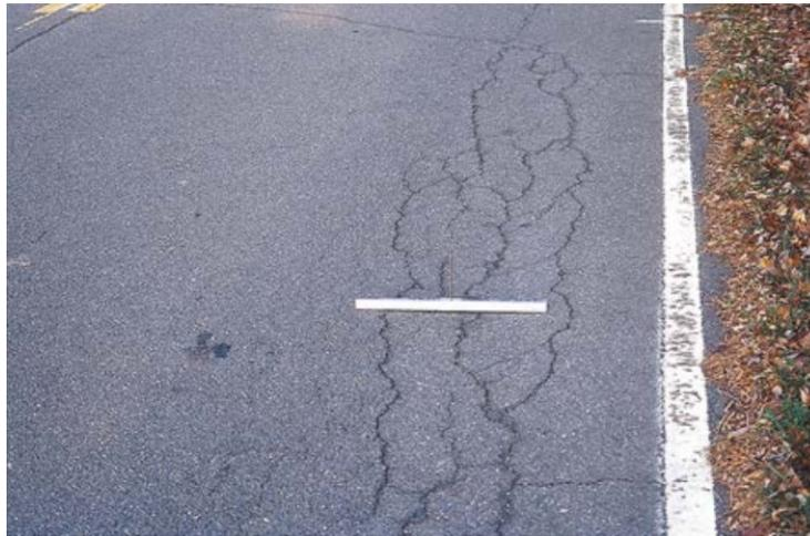
Figure 2.3: Example of fatigue cracks on pavement [21].
