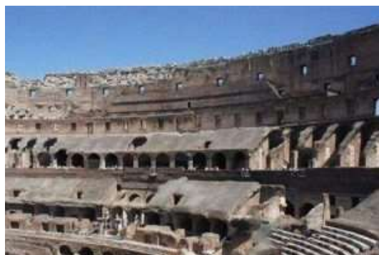
Figure 1 The Colosseum; its material was of travertine limestone, tuff (volcanic rock), and brick-faced concrete. @wikipedia
