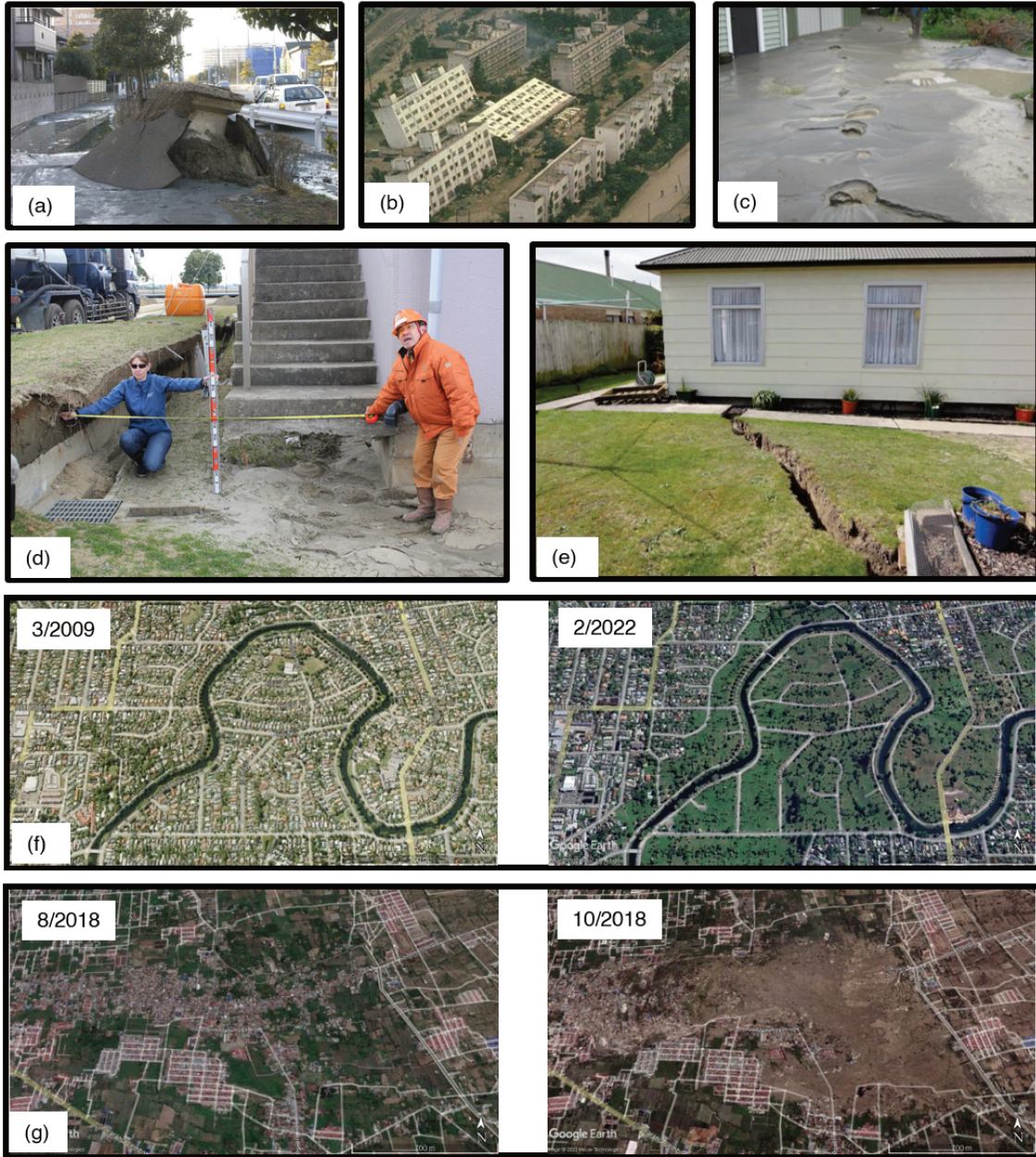
Figure 1: Liquefaction manifestations and damage. (a) floating of sewage manhole in Urayasu Japan; 2011 Great east Japan earthquake (photo from (Ishihara et al., 2011)) . (b) tilted buildings in Niigata, Japan; 1964 Niigata earthquake (photo from Wikipedia). (c) Sand blows (water escape features) in Christchurch, New Zealand; Canterbury earthquake sequence 2010-2011 (photo from (Quigley et al., 2013)). (d) Ground settlement in Kamisu, Japan; 2011 Great east Japan earthquake (photo from (Oregon State University, 2011)). (e) ground lateral spreading in the Christchurch area, New Zealand; 2010 Darfield earthquake (photo from (Cubrinovski et al., 2012b)). (f) a completely abandoned neighborhood, 11 years after the 2011 liquefaction event (Avonside, Christchurch New Zealand; Photos: Google Earth). (g) before and after a liquefaction event that initiated massive gentle-slope landslides in September 2018 in Palu, Indonesia (Photos: Google Earth).
