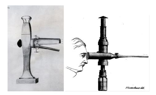
Figure 1.2: Early models of endoscopes. *Lichtleiter* by Bozzi (left) Endoscope by Desormeaux (right). Image adapated from [Desormeaux, 1865]
